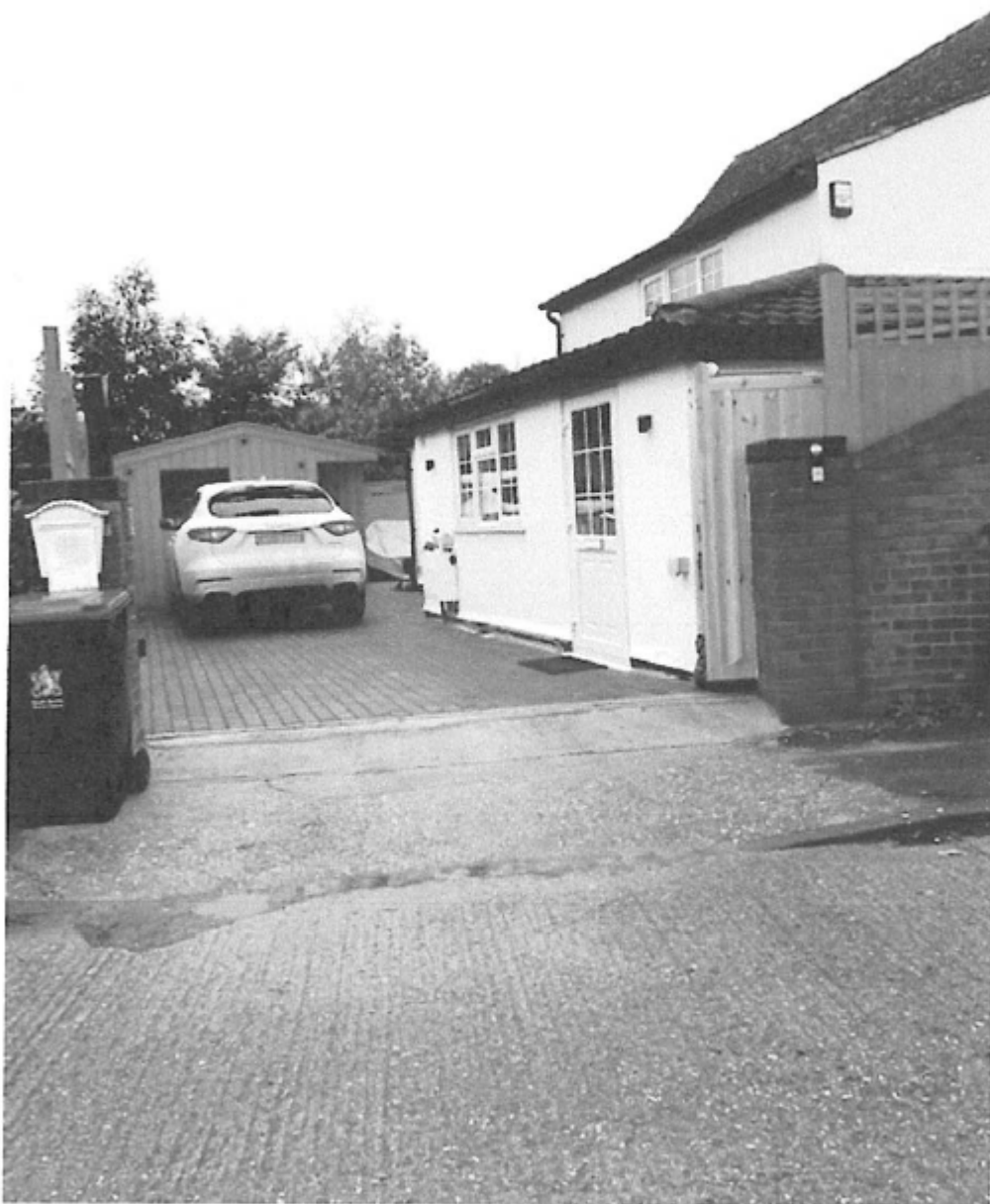
Entrance to 14 Mansion Lane within Iverdale Close. Structure behind parked vehicle subject of Licensing application.
